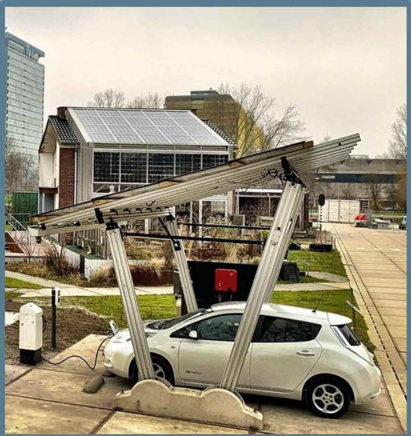
A solar carport with vehicle-to-grid (V2G) charging at the Green Village, TU Delft
