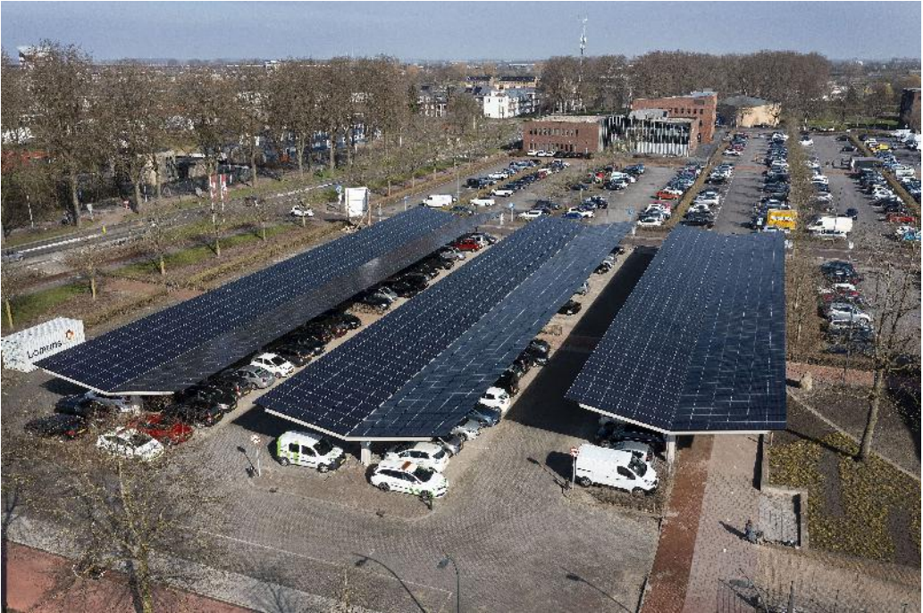
Figure 1.4: Solar carports for EV charging constructed at the municipality building, Dronten, the Netherlands
