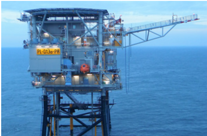
An existing oil and gas platform off the Dutch coast is being converted to the world's first offshore hydrogen platform. Electricity generated by offshore wind turbines will be used to convert seawater into demineralized water and to power a 1 MW electrolyser producing clean hydrogen.
