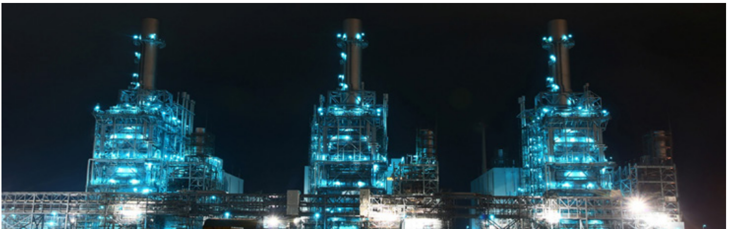
Near a crucial hub in the cross-border energy network connecting the Netherlands to Germany and Norway, Nuon/Vattenfall is preparing to convert an existing power plant to hydrogen. The first of the plant's three 440 MW units will run on (low-carbon) hydrogen by 2023. By converting the remaining units and switching to clean hydrogen by 2030, this is likely to become the world's first carbon-neutral hydrogen-fuelled power plant.
